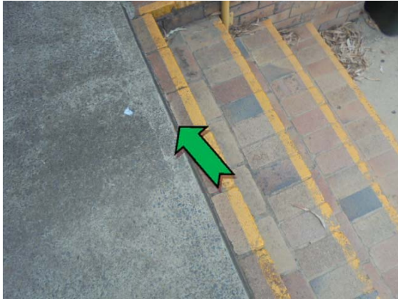
Photo 1. Exterior, entrance, expansion joint – non asbestos-containing bituminous material.
